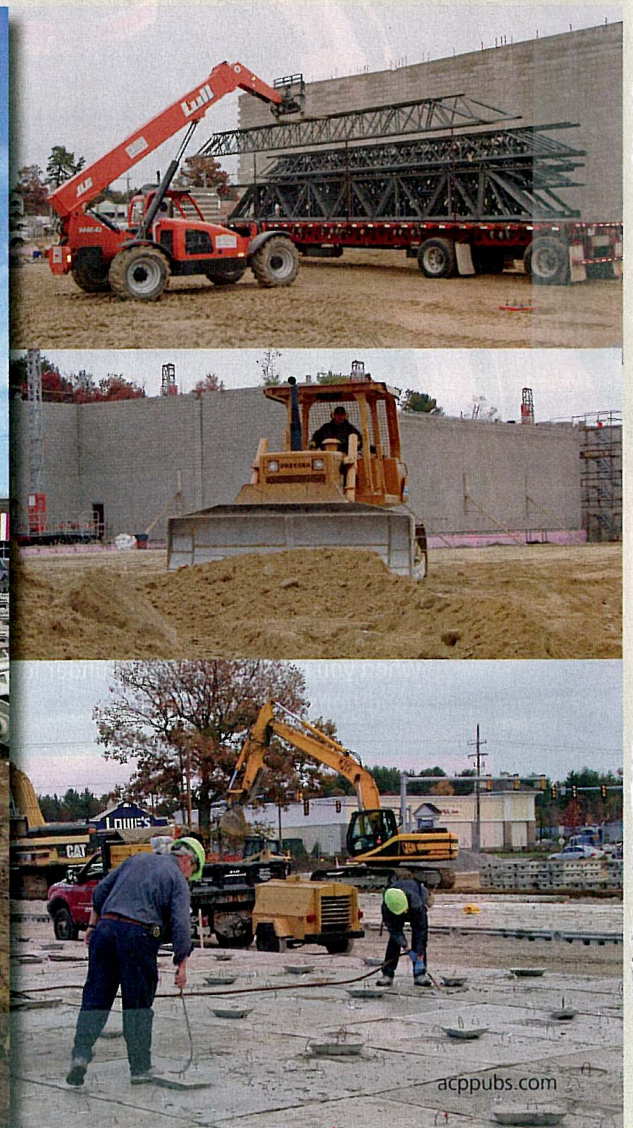
Middle right: HPB Construction’s Dresser TD15E dozer rough grades gravel for parking lot.
