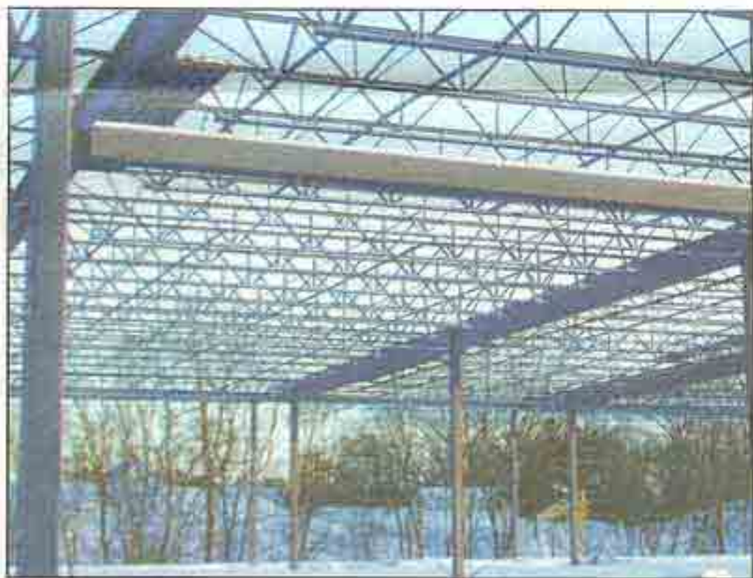
A Jay Steel project in progress. Courtesy of Jay Steel.
